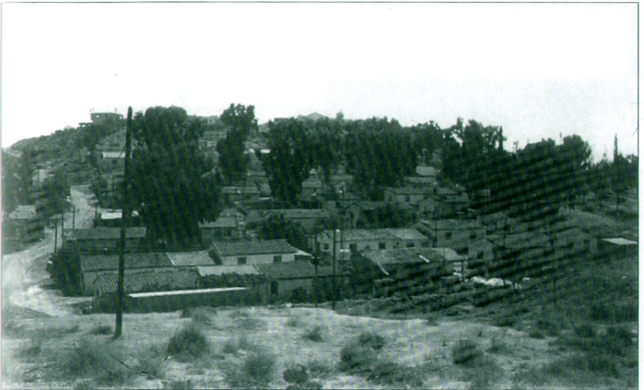
Fig. 5: Cyprus — General view of CMC Houses in Lefke.
