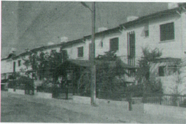
Fig. 14. The view of the row-type social housing complex in Gazimagusa (Famagusta).
