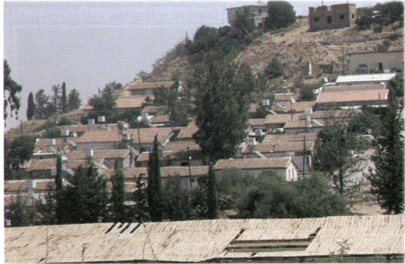
Figure 2. CMC housing district from British period in Lefke (Hoşkara and Zafer, 2005).
